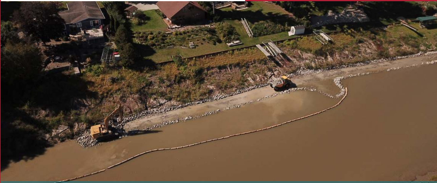
The beginning stages of shoreline stabilization along Sanford Lake. This was necessary due to severe erosion after the lake levels dropped.
