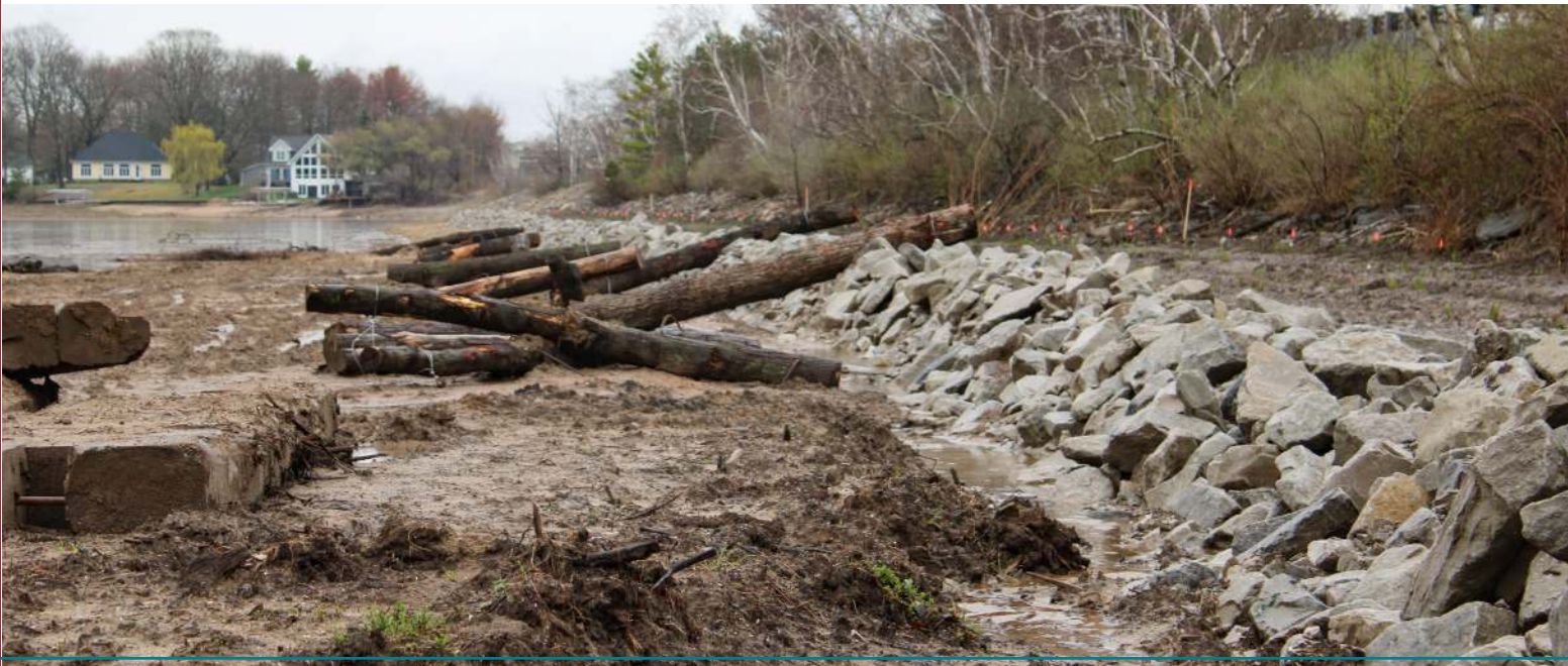
Fish habitat was installed throughout the lake prior to refilling.
