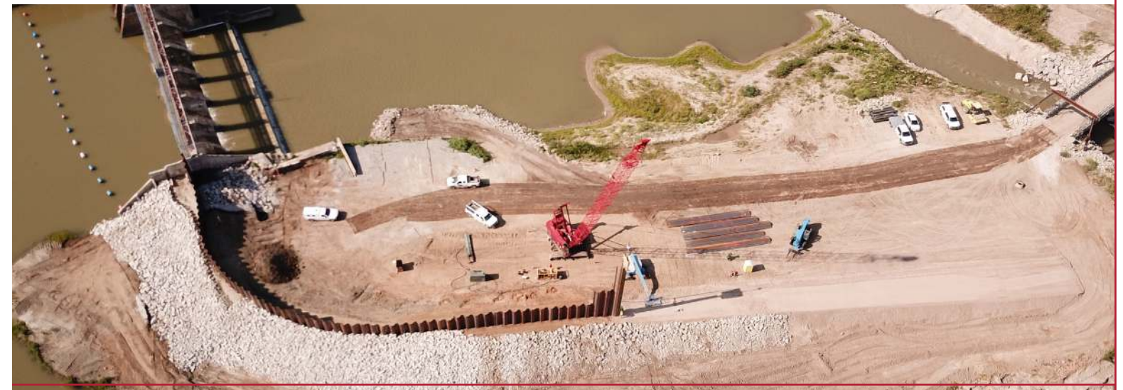
Work completed along the shoreline of Sanford Lake in 2022 as part of the interim stabilization project to reduce erosion and continued damage.
