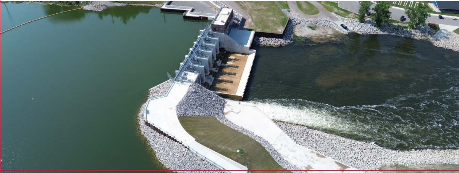
Sanford Dam after lake refill
